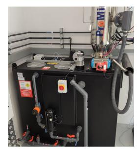
ProMinents Pro Sat - Vac Fluoride Saturator System. Provides a safe & economic way of dosing fluoride into your water supply with ProMinents Vacuum Loading System. To ensure dust free loading of 25kg sodium fluoride bags.
